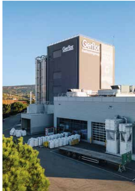
↑ Usine LVT, Saint-Paul-Trois-Châteaux, France.
